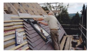
The solar water heating tubes were installed whilst the scaffolding was still in place and before the last rows of tiles were fixed. The rainwater gutters were also installed before the scaffolding was removed.
