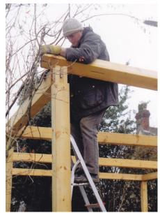
The Flat is based upon a standard Beamlock 4-bay kit of posts and beams, bay 4 forming the entrance to the Flat with the bathroom behind. The three other bays are open-fronted for the car, ride-on mower, log storage etc. The central heating boiler and electricity switchboard are in a cupboard at the back of bay 3.
