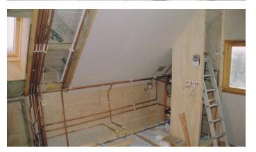
Mixer valves were installed on the bathroom hot water supply to ensure that no-one could be scalded by the potentially very high temperatures reached by the solar water heating.
