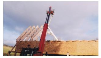
roof trusses are very strongly constructed to prevent spreading under the weight of the tiles so that the upstairs headroom in the Flat is not obstructed by tie beams. Hence the need for calculations by the structural engineer.
