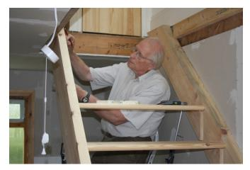
The staircase was assembled in situ with the treads and risers glued and wedged into the strings. Then it was possible to build the upstairs ballustrade and the plywood wall between the stairs and the hall and bathroom.
