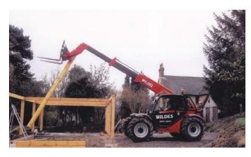
Diagonal braces were installed at several of the junctions of post and beam, according to Beamlock's plans. These require slots to be routered to take the metal ends of the braces and holes drilled for metal pegs to be hammered into the braces. A plastic template was supplied for this work. A good router is needed, plus a long bit (obtainable from the Beamlock suppliers). Installing these braces and lining up the holes for the metal pegs was the most tricky part of the Beamlock construction.
