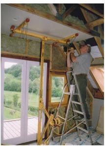
Now that the building was watertight, the floor panels were installed and work began on installing cabling for lighting and power points. Once these were in situ, insulation was placed in the wall and ceiling voids and plasterboard fixed, starting at the bedroom end. A panel
